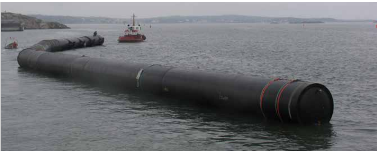
FIGURE 4.21: STRUCTURED WALL PE-HD FLOATING SYSTEM
